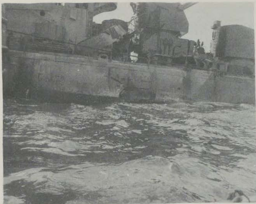
Photo 1: Port side in way of damage. Ship has starboard list.
