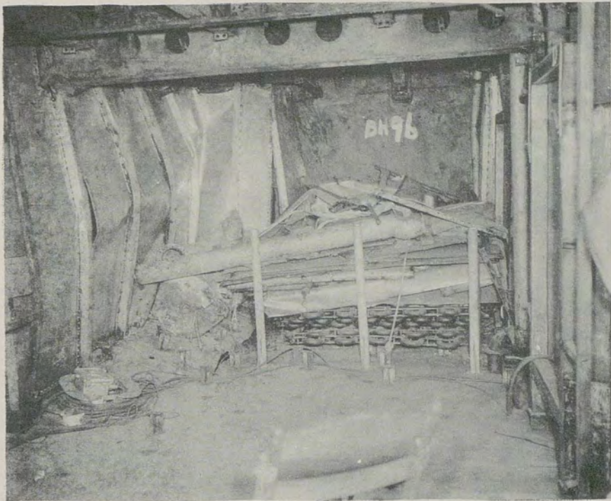
Photo 11: Looking forward in C-307-6A showing damaged bulkheads and torn deck plating.
