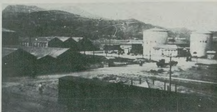
FIGURE IX - 43. Takao. Mitsubishi petroleum storage facility.
