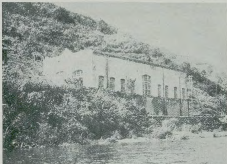
FIGURE IX - 52. Taihoku-shū. Kizan hydro plant.
