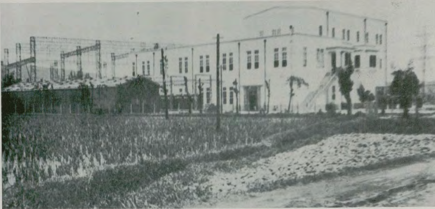
FIGURE IX - 71. Takao. Switching station at S terminus of 154 kv transmission line S from Jitsugetsu-tan hydro development.
