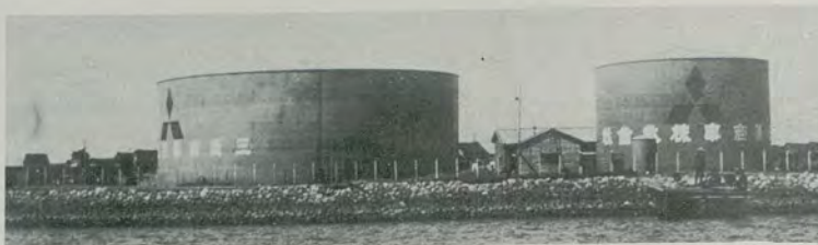
FIGURE IX - 42. Takao. Mitsubishi petroleum storage facility near harbor.
