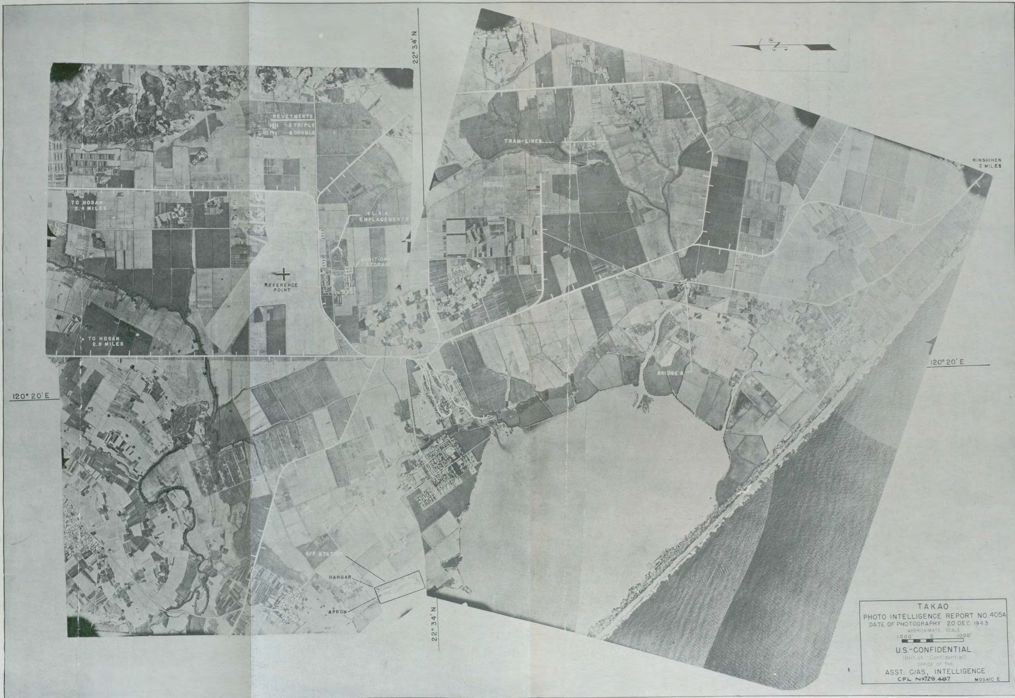
FIGURE XIII - 18. Reigaryō-Takao Harbor. Heavy bomber landing ground and seaplane station.
